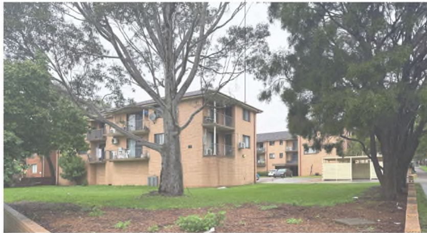
150 The Boulevard, Punchbowl, building to be demolished
