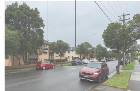
150 The Boulevard, Punchbowl, building to be demolished
