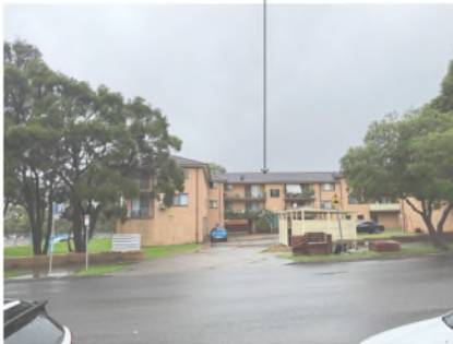
150 The Boulevard, Punchbowl, building to be demolished
